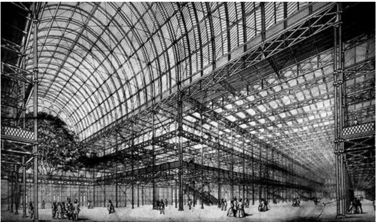
Crystal Palace structure
