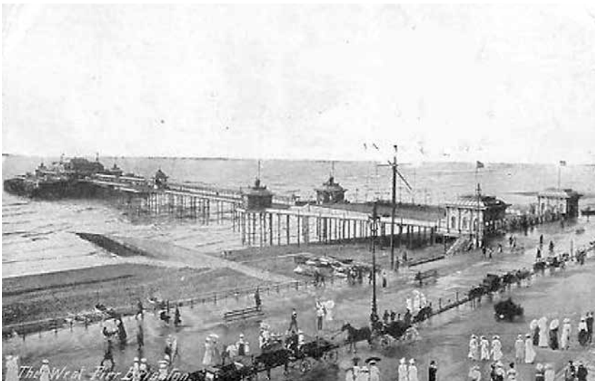
West pier Brighton, 1866
