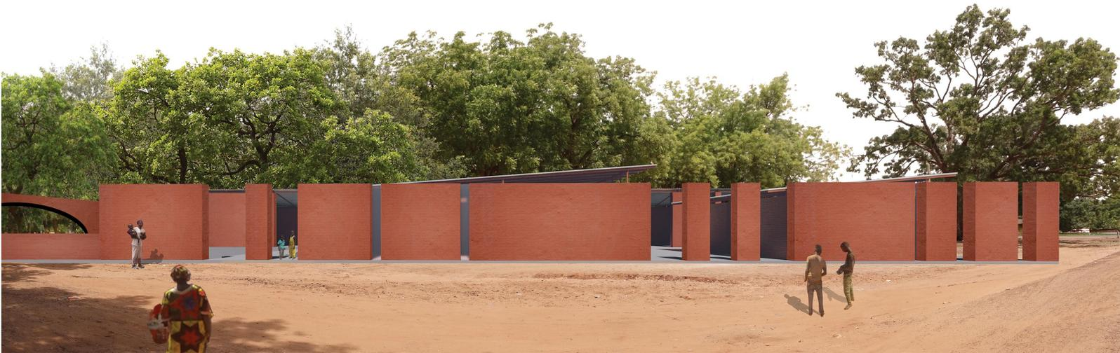
The roof is raised to allow ventilation and lighting of the space below.
