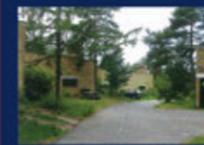
Prog. Kingo Housing Loc. Helsingor, Danimarca arch. Jørn Utzon
